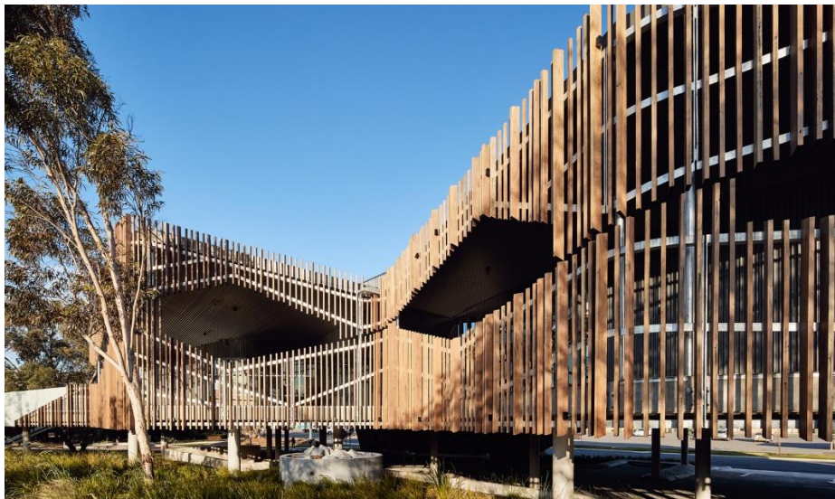
Timber paneling on façade at Centre for Nyoongar Culture and Environmental Design (iredale pedersen hook architect)
