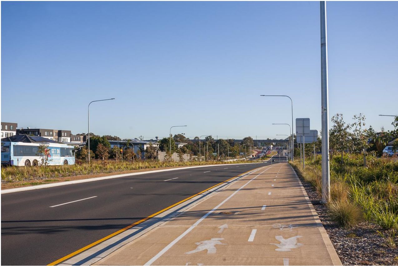
View 7_MG_7935 – Existing
