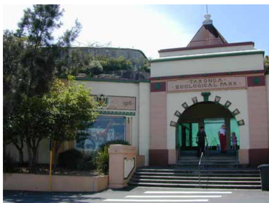
Figure 7.17 Lower Entrance Building front facade.
