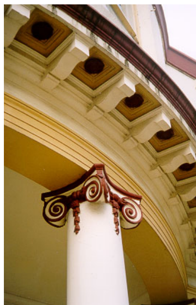
Figure 7.13 Upper Entrance Building detail of rear facade.
