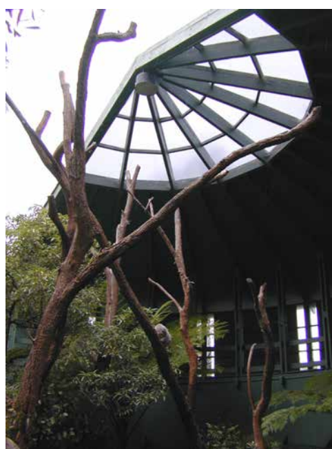
Figure 7.24 Internal view of the Koala House.
