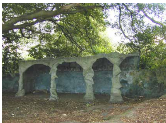
Figure 7.48 The grotto effect applied to the supports of the Deer Shelter.
