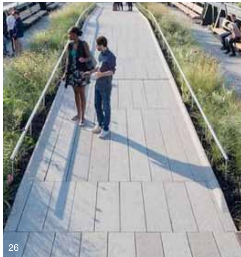
Image 26: Concrete pavers and planks on raised footings create a textured pathway within the African Waterhole Pavillion.
