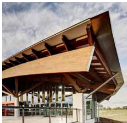
Image 16: Timber glulam structures span across the Giraffe House, providing shade and
