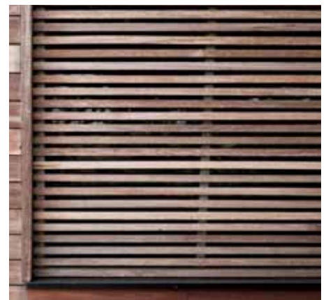
Image 17: Timber screen walls provide natural textures and soft back drop to the Savannah
