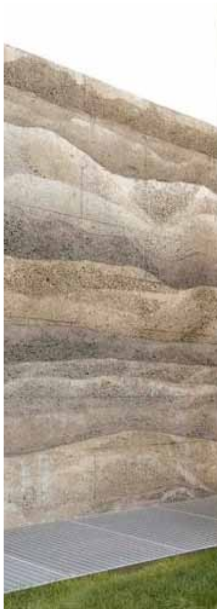
Image 30: Rammed earth walls to all Congo Viewing shelters.
