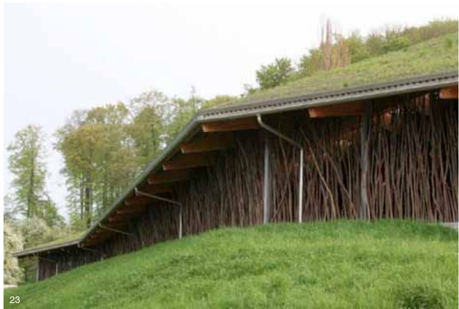
Image 23: The Meerkat Back of House has a Green roof on lightweight structure. The green roof and organic wickerwork walls allow the architecture to recede into the landscape and exhibit.
