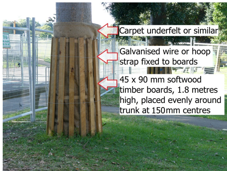
Figure 3 – Detail of Trunk Protection
