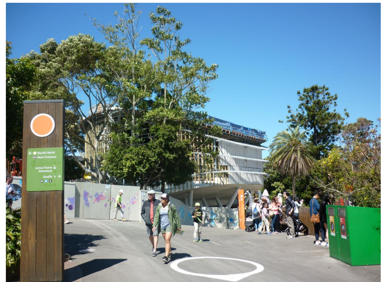
Photo 3.1 The Centenary Theatre under construction in the area adjacent to the northern part of the project site.
