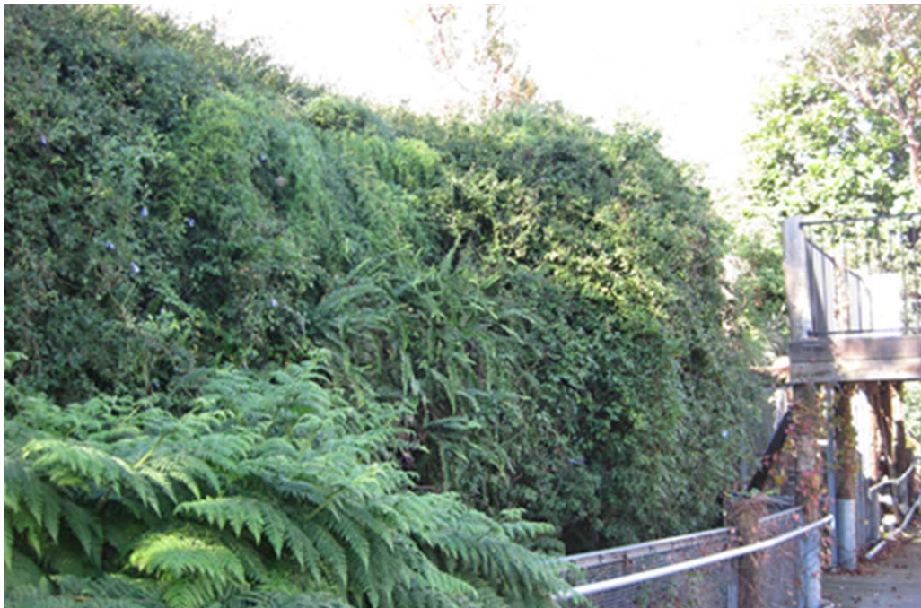
Photo 14 – Sandstone and possibly retaining wall cliff covered with vegetation
