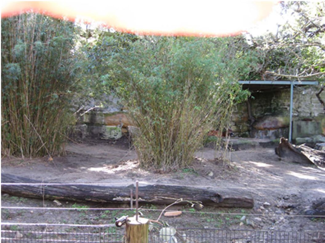
Photo 7 – Rock outcrop, block retaining wall, shotcrete in Bongo enclosure
