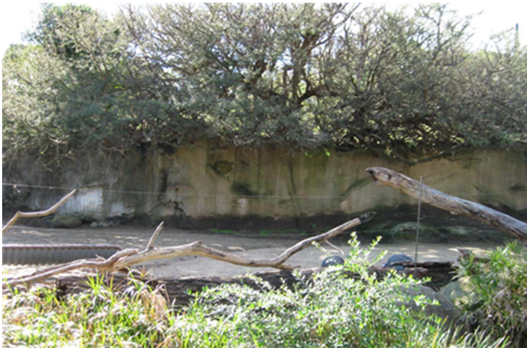
Photo 8 – Shotcrete and sandstone in Zebra enclosure
