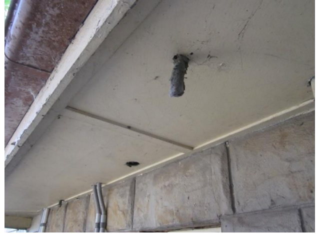
Photo 2 Turner House – AC eaves
