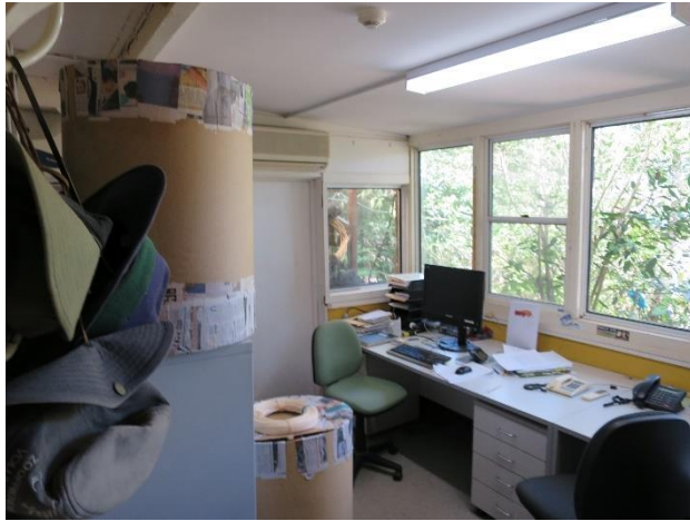
Photo 1 Turner House front office – AC walls and ceiling
