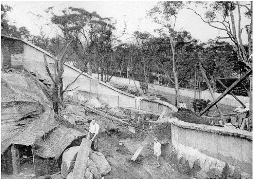
Figure 3.5 The construction of one of the circular monkey pits, c1915. Note the natural bushland in the background (Taronga Zoo Archives).
