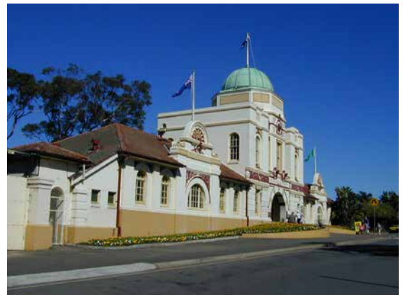
Figure 2.5 Upper Entrance building.
