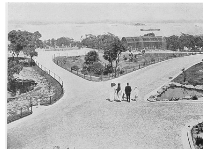
Figure 4.3 View overlooking site and from top entrance building – 1916.
