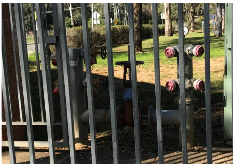
150mm 4 Point Fire Hydrant Booster Assembly
