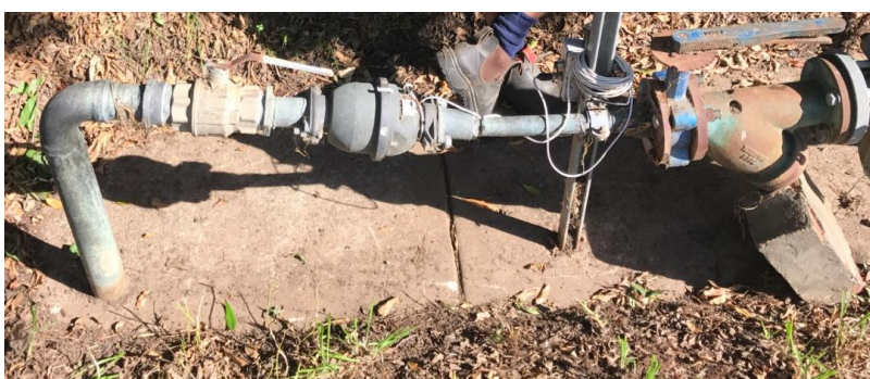
Master Cold Water Meter & RPZD Devices
