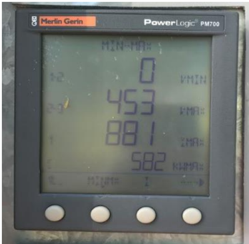
Sub-meter reading within the MSB
