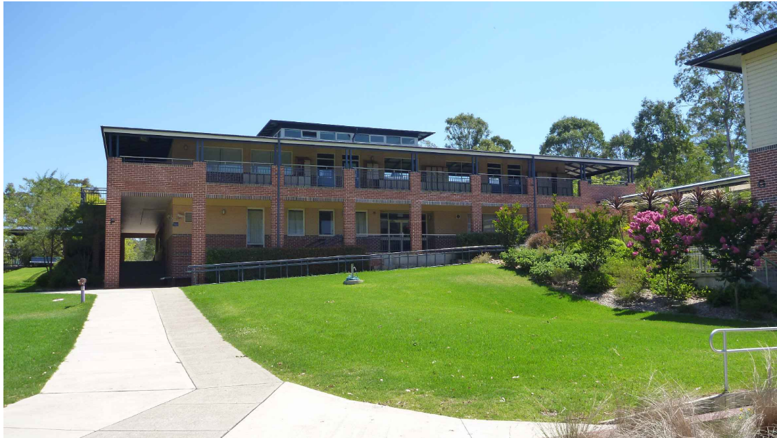
VIEW 2: VIEW OF TYPICAL SENIOR MODULES
