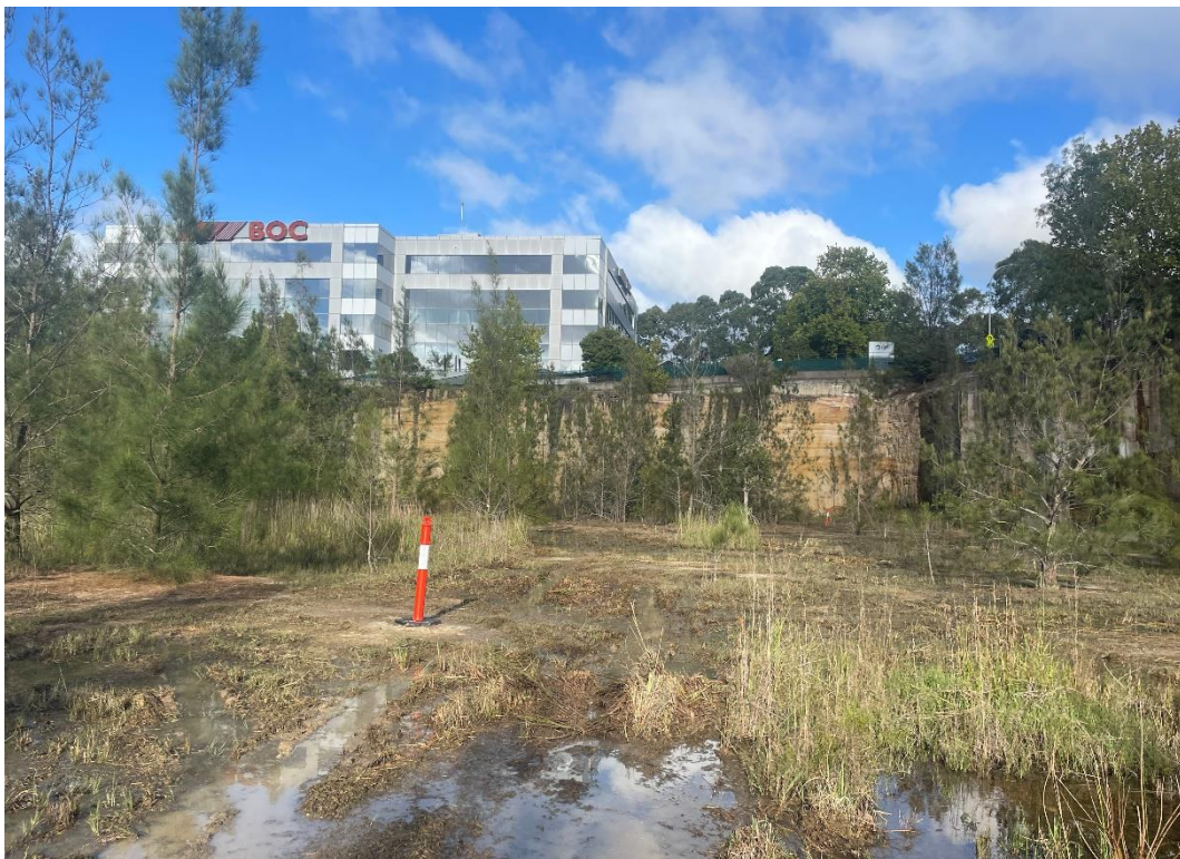
Photo 2: Sandstone cutting Facing West
