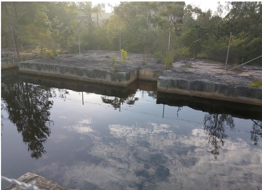
Photo 4: Dam Within Sandstone Cut
