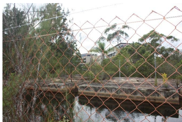
Figure 3.4 Deep excavation within the northern portion of the study area, facing east towards the heritage cottage at 2 Richardson Place.
