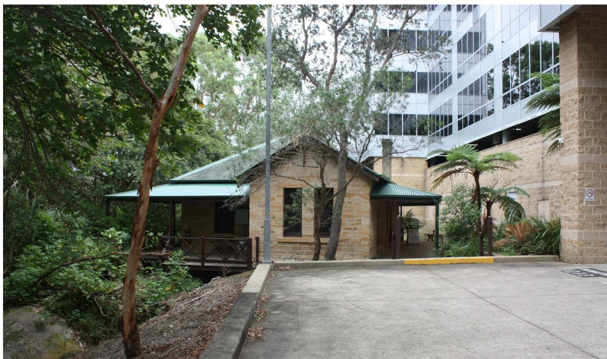
Figure 4.1 The heritage listed cottage at 2 Richardson Place, looking towards the study area. The Honeywell office building is to the right of the image. (Source: GML 2025)
