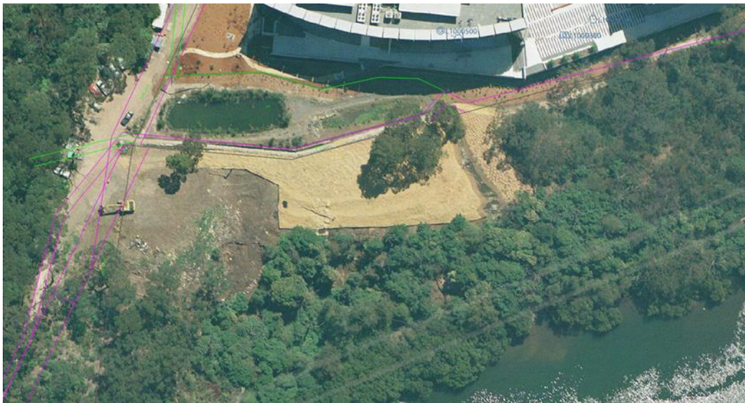
Figure 6-2: Existing Drainage Infrastructure Imagery-SW Corner (Source: CoR Council Drainage Officer-Council Correspondence)
