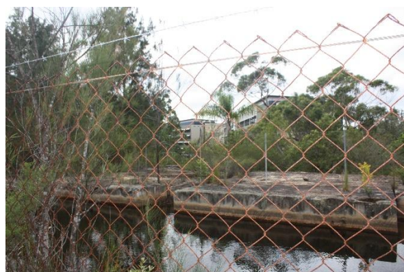
Figure 4.5 Deep excavation within the north of the study area, facing east towards the heritage cottage at 2 Richardson Place.
