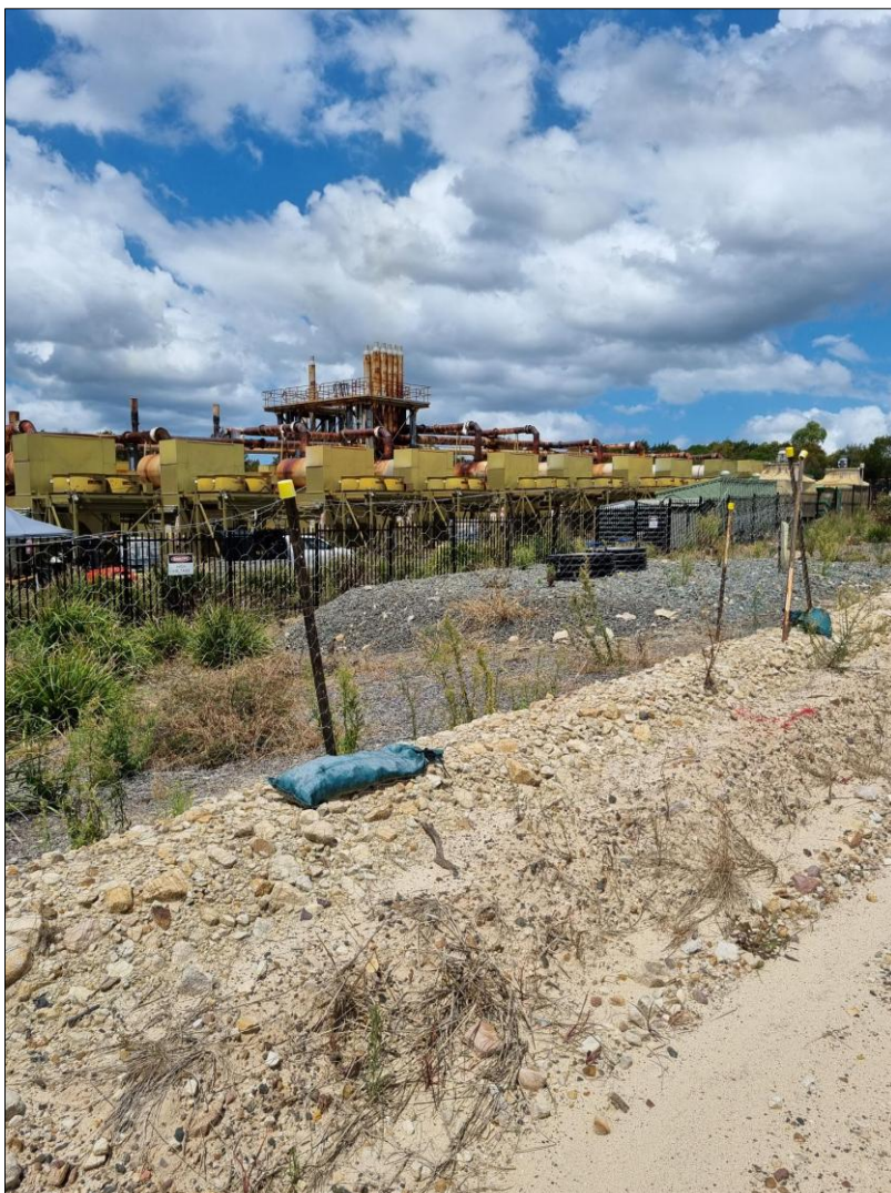
Figure 7.1 Viewpoint of the existing power station from within the LHRRP looking east
