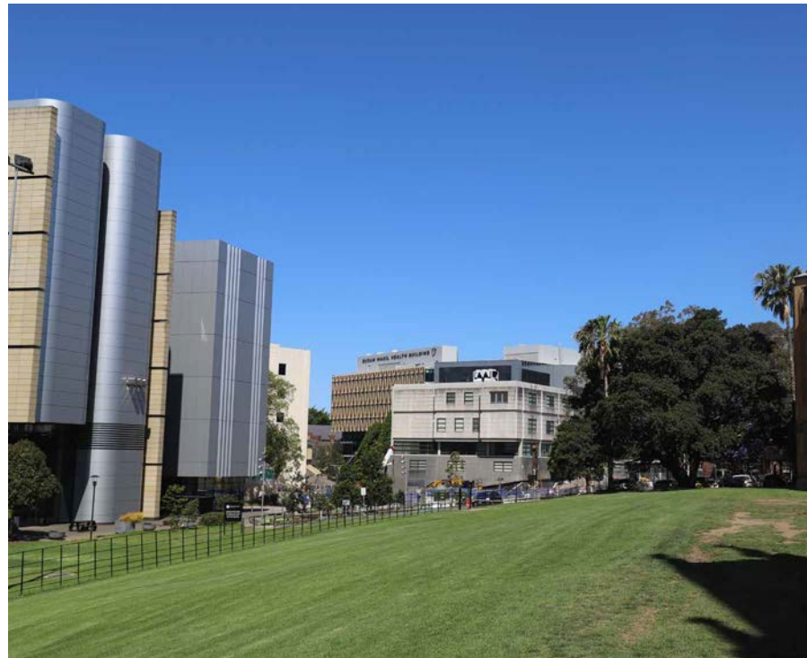
Photo 7. South-east view from northern corner of the main building.
