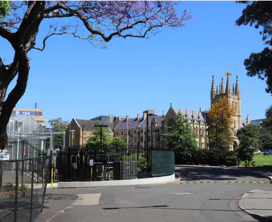
Photo 2. View from Parramatta Road at Orphan School Creek Lane (CMP View 4b).
