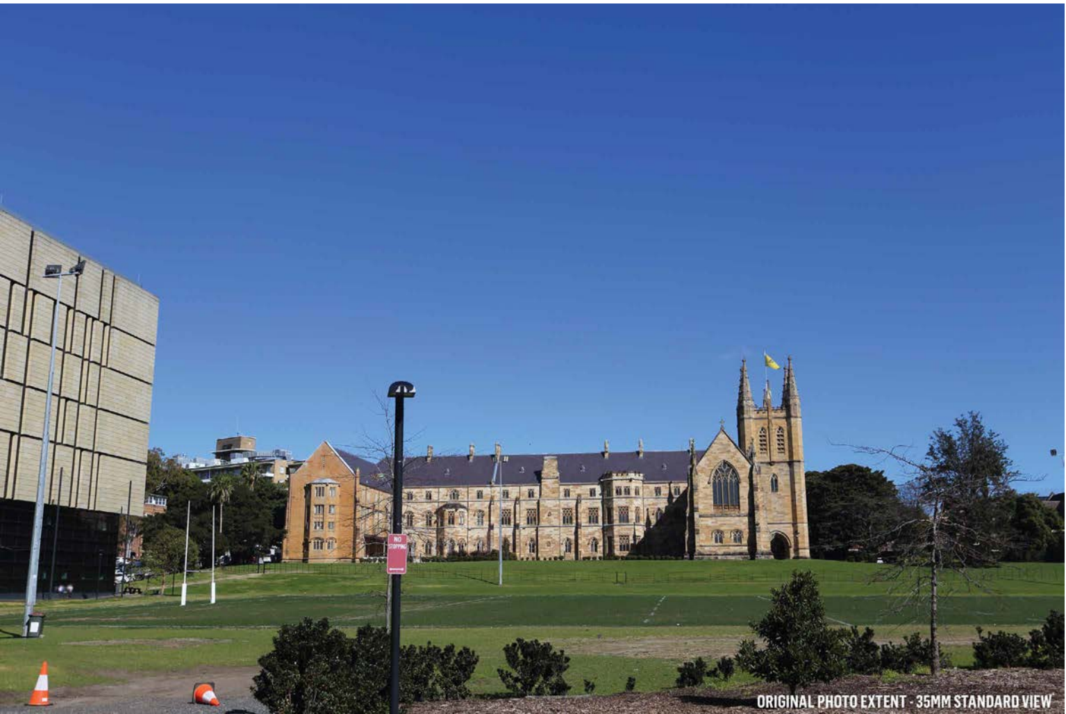
Figure 17 Viewpoint 03 existing view.
