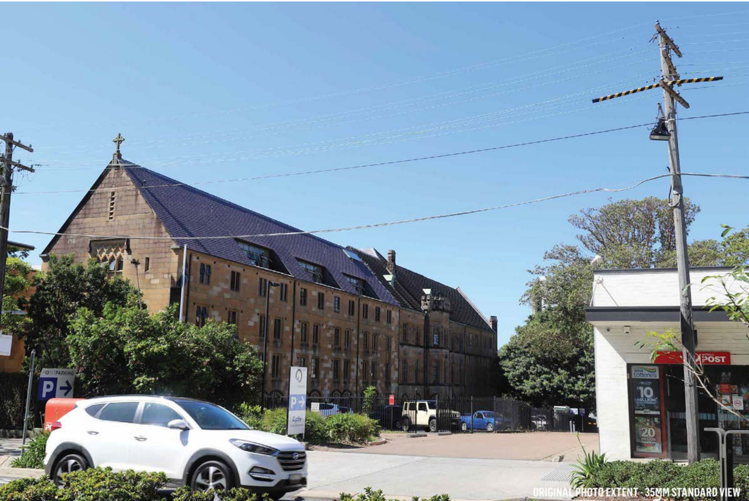
Figure 26 Viewpoint 06 existing view.
