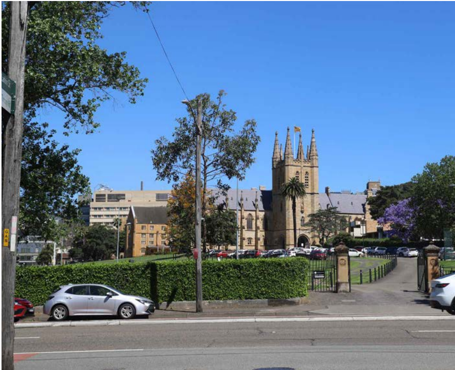
Photo 1. View of Freehill Tower southward along Larkin Street (CMP View 3)
