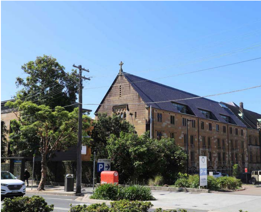
Photo 13. Freehill Tower seen from Missenden Road looking northward ( CMP View 1 ).
