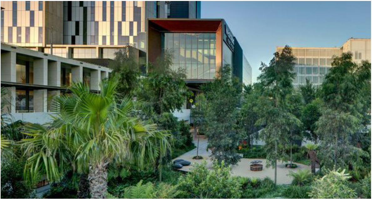
Westmead Hospital Central Acute Services Building
