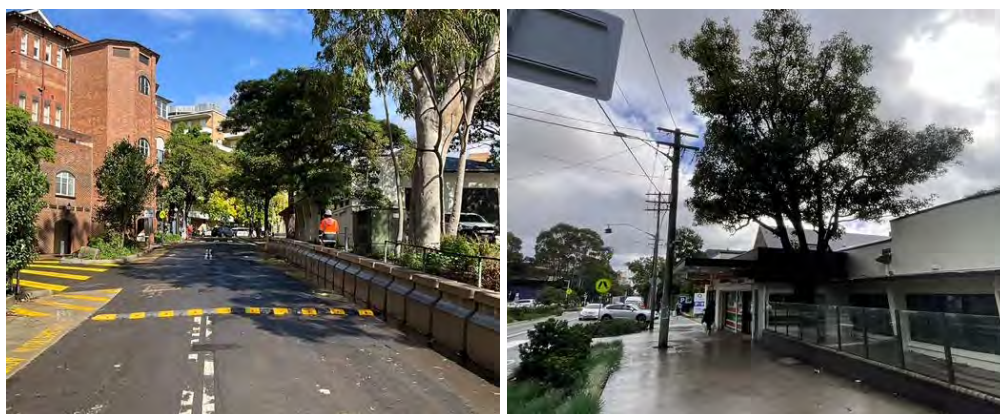
Figures 14 & 15: The John Hopkins Drive frontage (Left) and the Missenden Road Frontage (Right) can be observed. (Source: Austin 28 th of April 2025)
