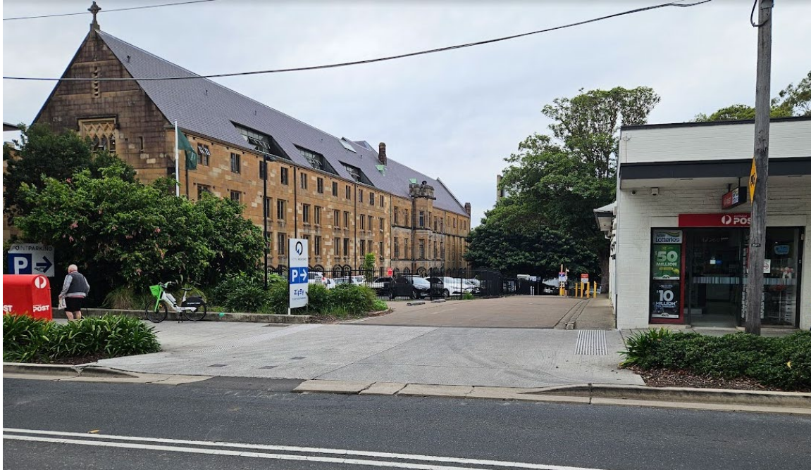
Figure 4 Existing vehicle access via Missenden Road
