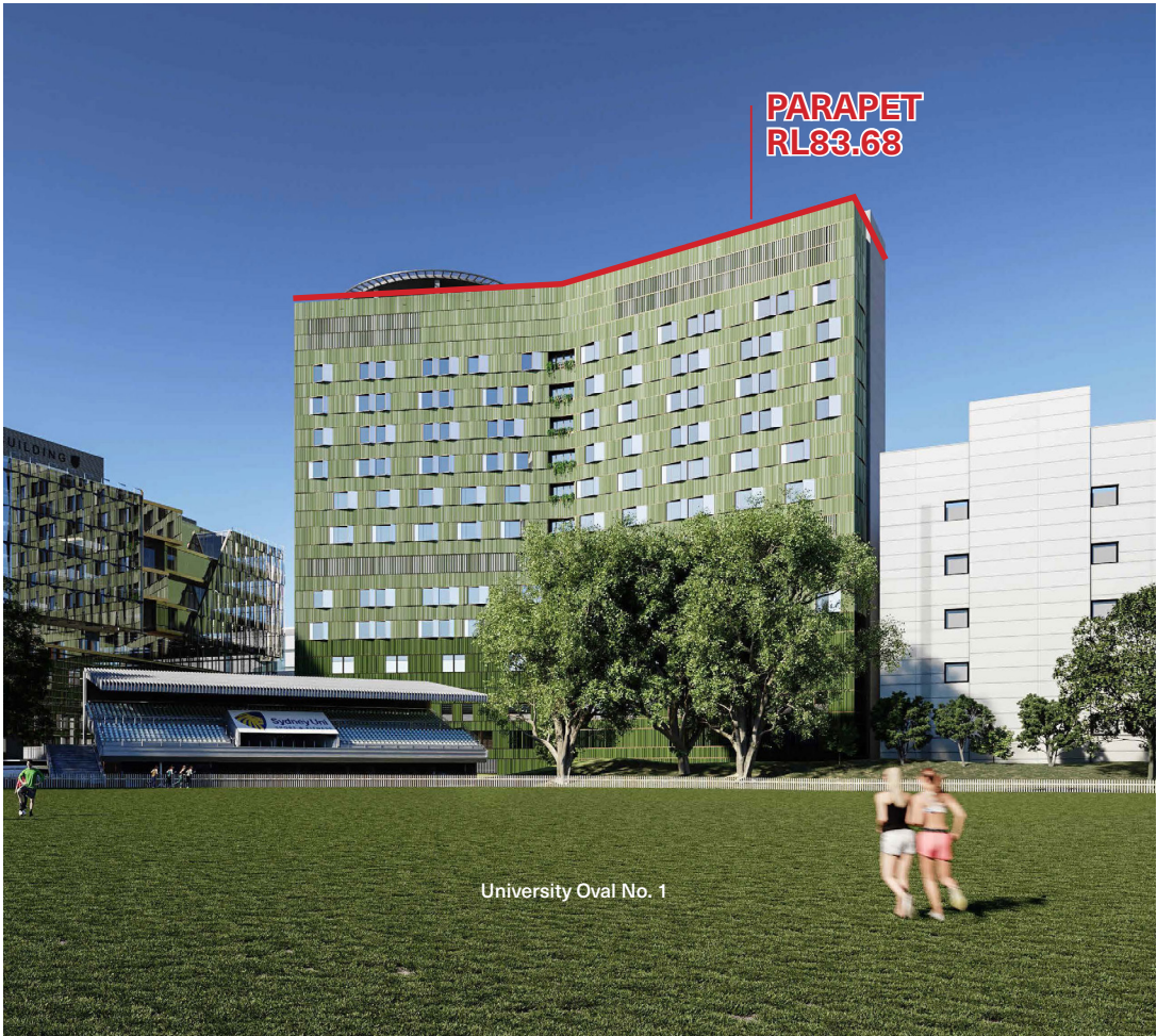
RPAH East Wing with University Oval No. 1 in the foreground with parapet height annotated [Source: RPAH Redevelopment Design Report - Jacobs, Bates Smart, Neeson Murcutt and Neille]
