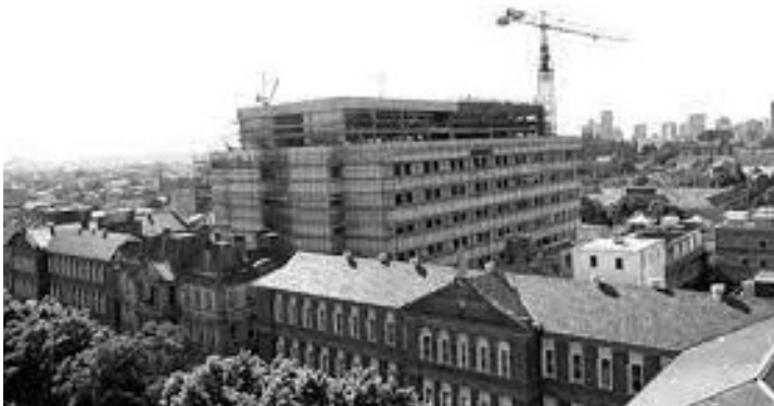
E Block under construction behind Albert Wing, Admin Block and Victoria Wing
