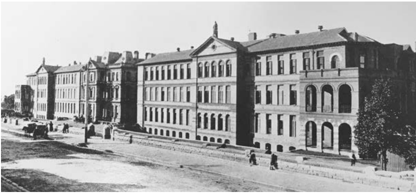
Royal Prince Alfred Hospital Albert Wing, Admin Block and Victoria Wing
