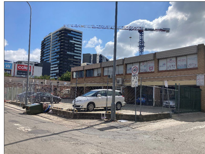
Photograph 8 – West View: West Elevation of Block 229-239 Pitt St
