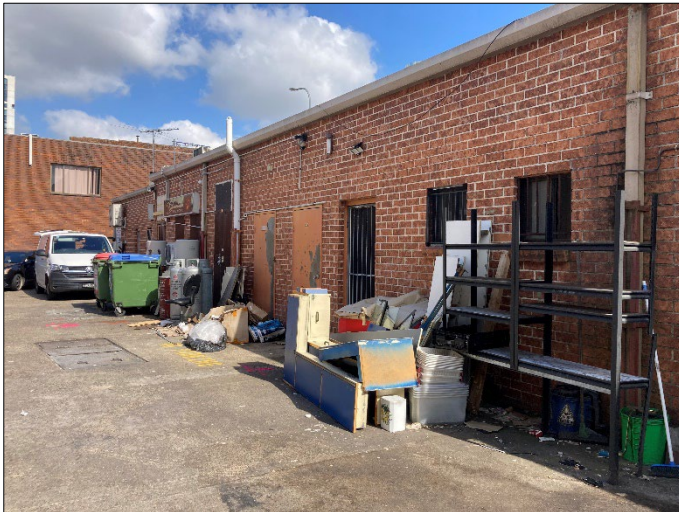
Photograph 3 – Rear View: Rear Elevation of Block 215 Pitt St
