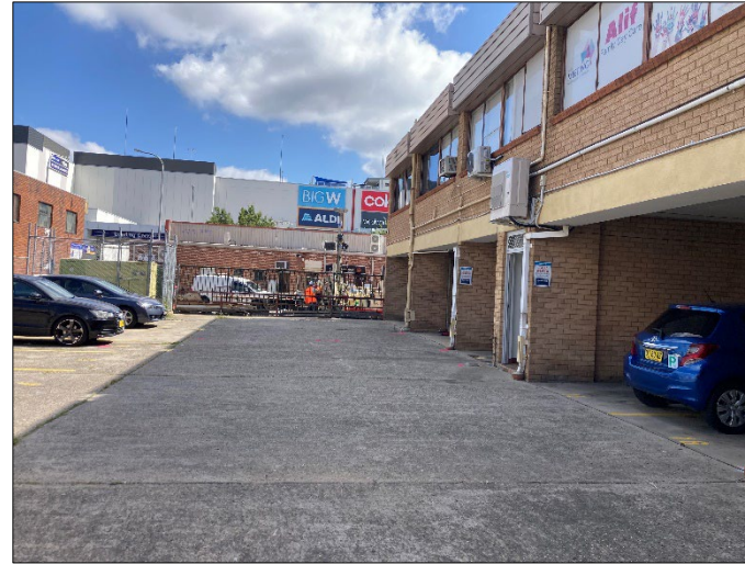
Photograph 10 – Rear View: Rear Elevation of Block 229-239 Pitt St
