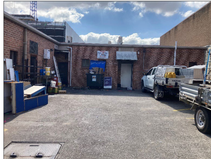
Photograph 4 – Rear View: Rear Parking of Block 215 Pitt St
