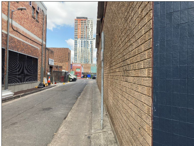
Photograph 7 – South View: South Elevation of Block 229-239 Pitt St
