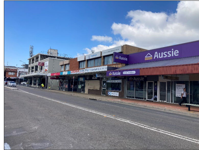
Photograph 6 – East View: East Elevation of Block 229-239 Pitt St
