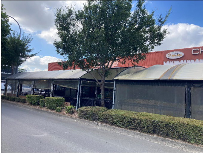
Photograph 1 – North View: North Elevation of Block 215 Pitt St
