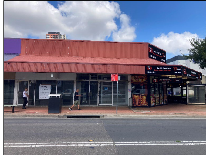
Photograph 2 – East View: East Elevation of Block 215 Pitt St
