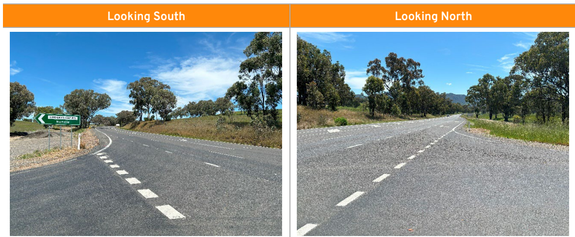
Figure 5: New England Highway and Lindsays Gap Road Intersection Photographs
