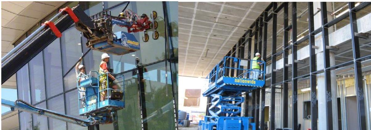
Figure 17: Glazed cladding being installed using a mobile crane and vacuum sucker units
