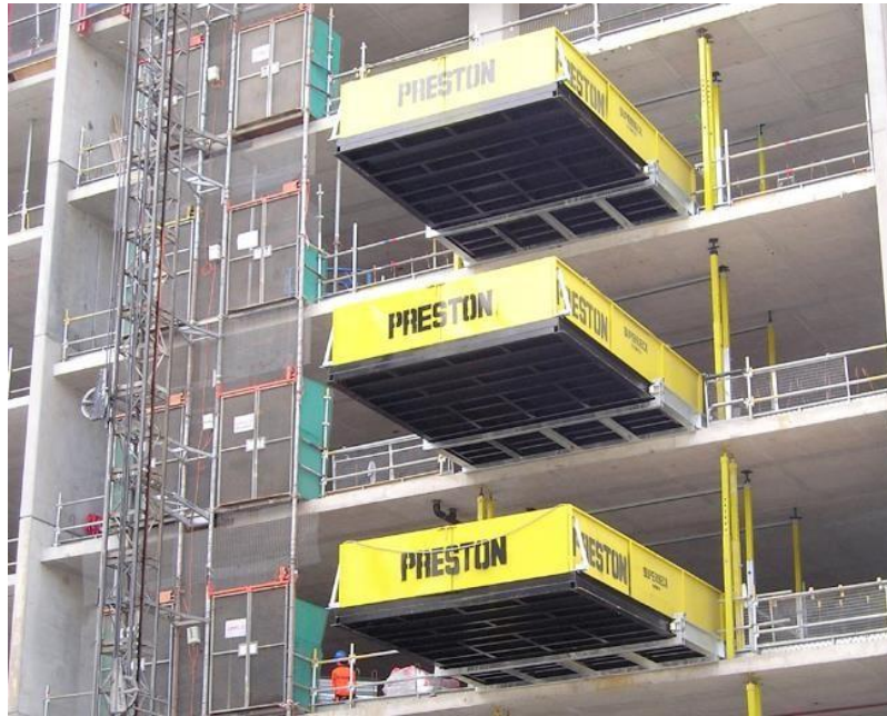
Figure 19: Example of loading decks
