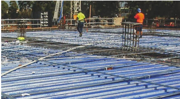
Figure 13: Kingflor-KF57 in use & Typical laying sequence of Kingflor-KF57
