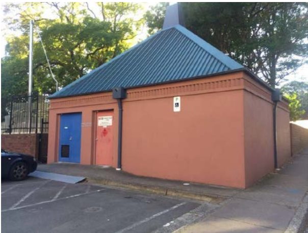
Picture 6 – Dangerous Goods Store (Northern Elevation)
