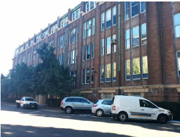
Picture 4 – Blackburn Building (Eastern Elevation)
