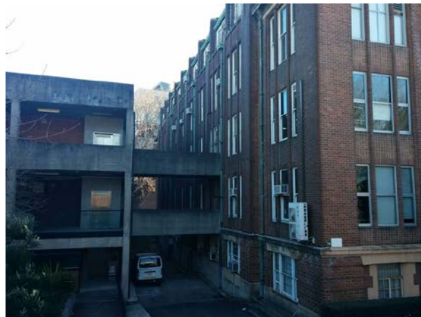
Picture 5 – Blackburn Building (Southern Elevation) and Bosch 1B Building
