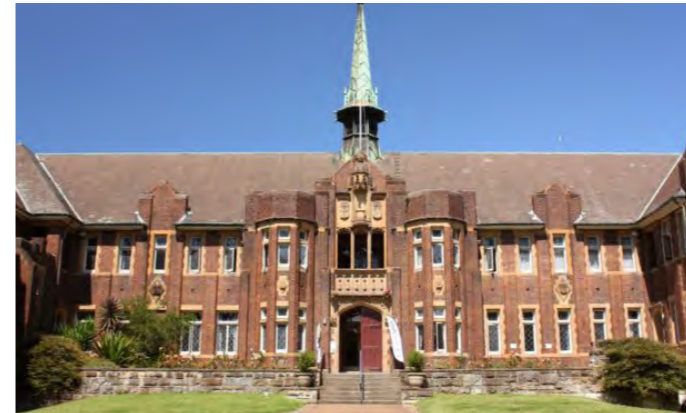
Stage 2 building faces Wesley College to the east across Western Ave.
