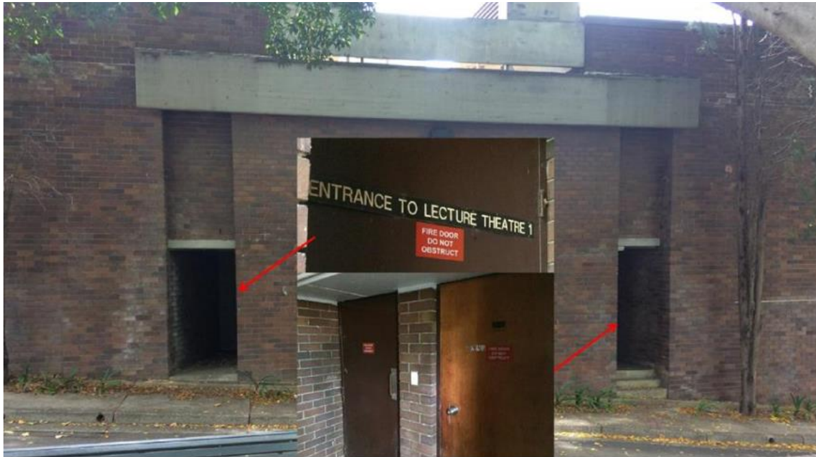
Figure 5: Fire exit doors in Bosch Building 1A to remain operational
