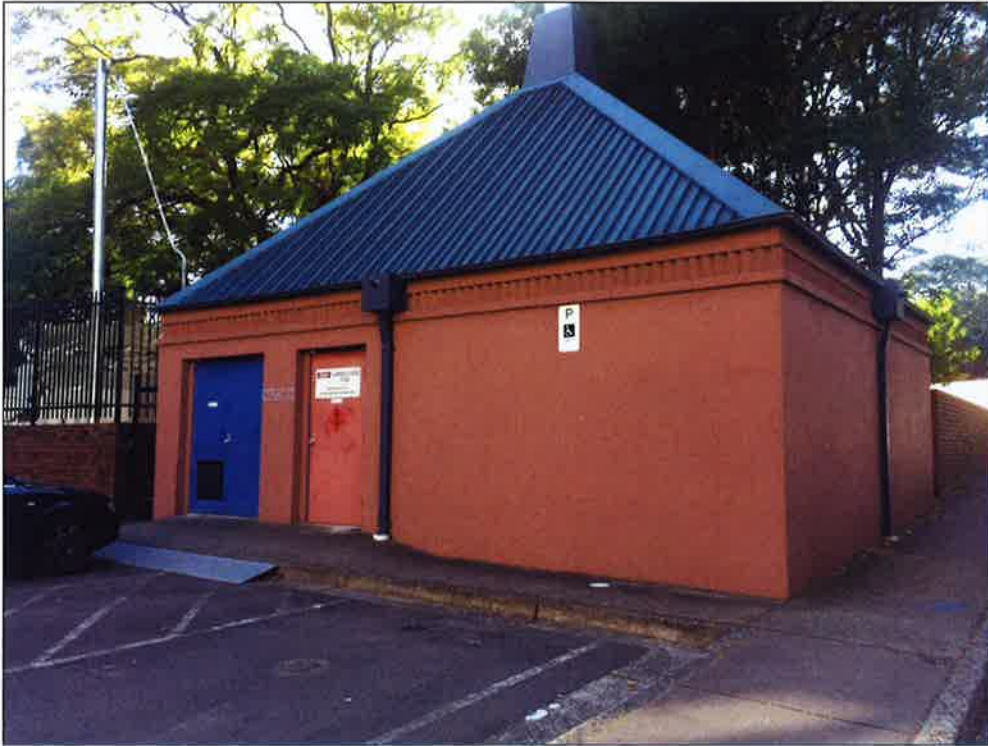
Image 3: Dangerous Goods Store (Northern Elevation)
