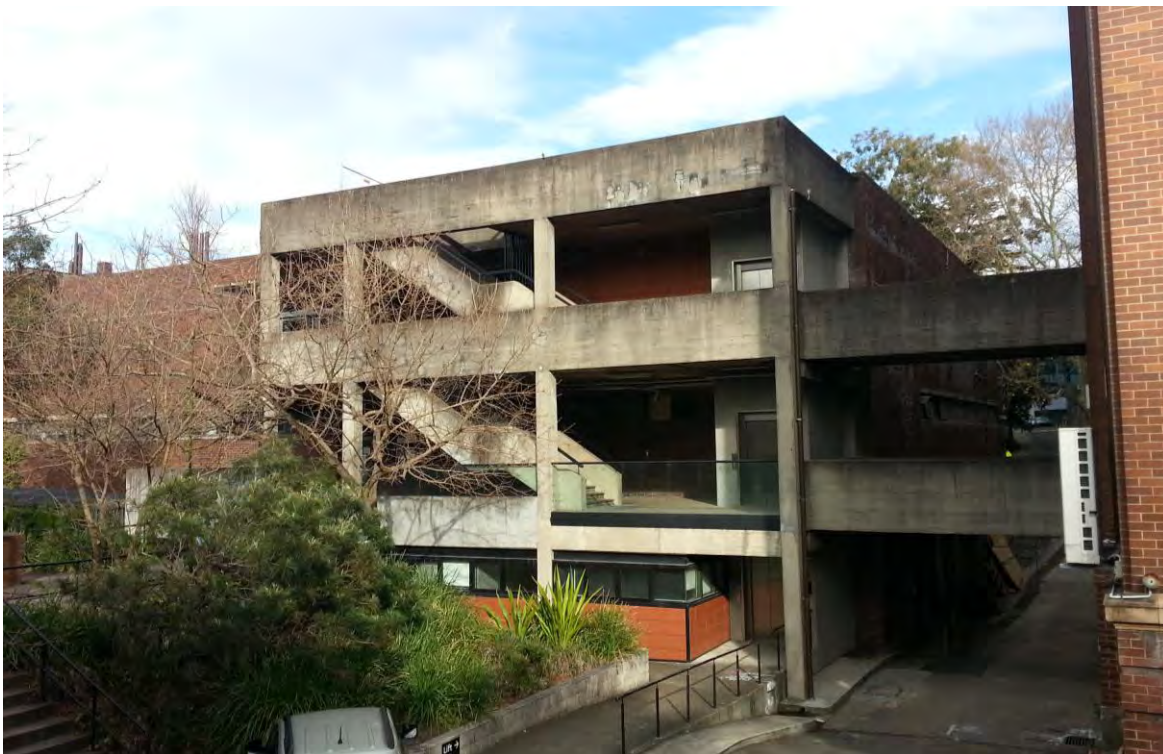
Figure 6.10 Eastern Elevation of Bosch 1B Building (D05), adjacent to the Blackburn Building (right) (source: Author, July 2017)
