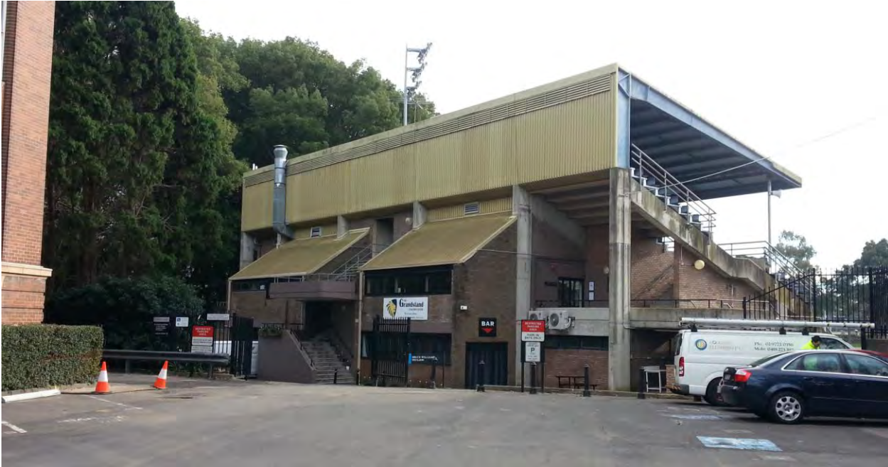
Figure 6.11 Oval No.1 Grandstand, backing on to the SWAOHB site (Blackburn Building, left) (source: Author, July 2017)
