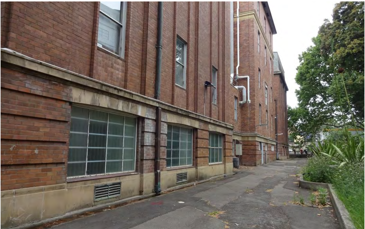
Figure 4 – View of the northern elevation, facing west
