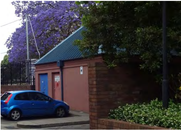
Picture 17 – View of the western façade of the building, facing north
