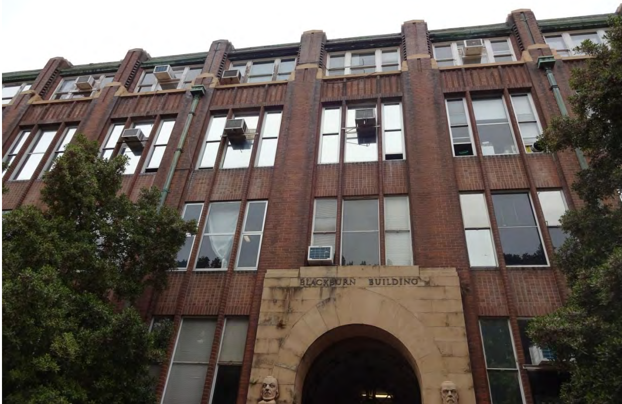
Figure 2 – Principal (eastern) façade of the building showing main entryway (Urbis 2016)
