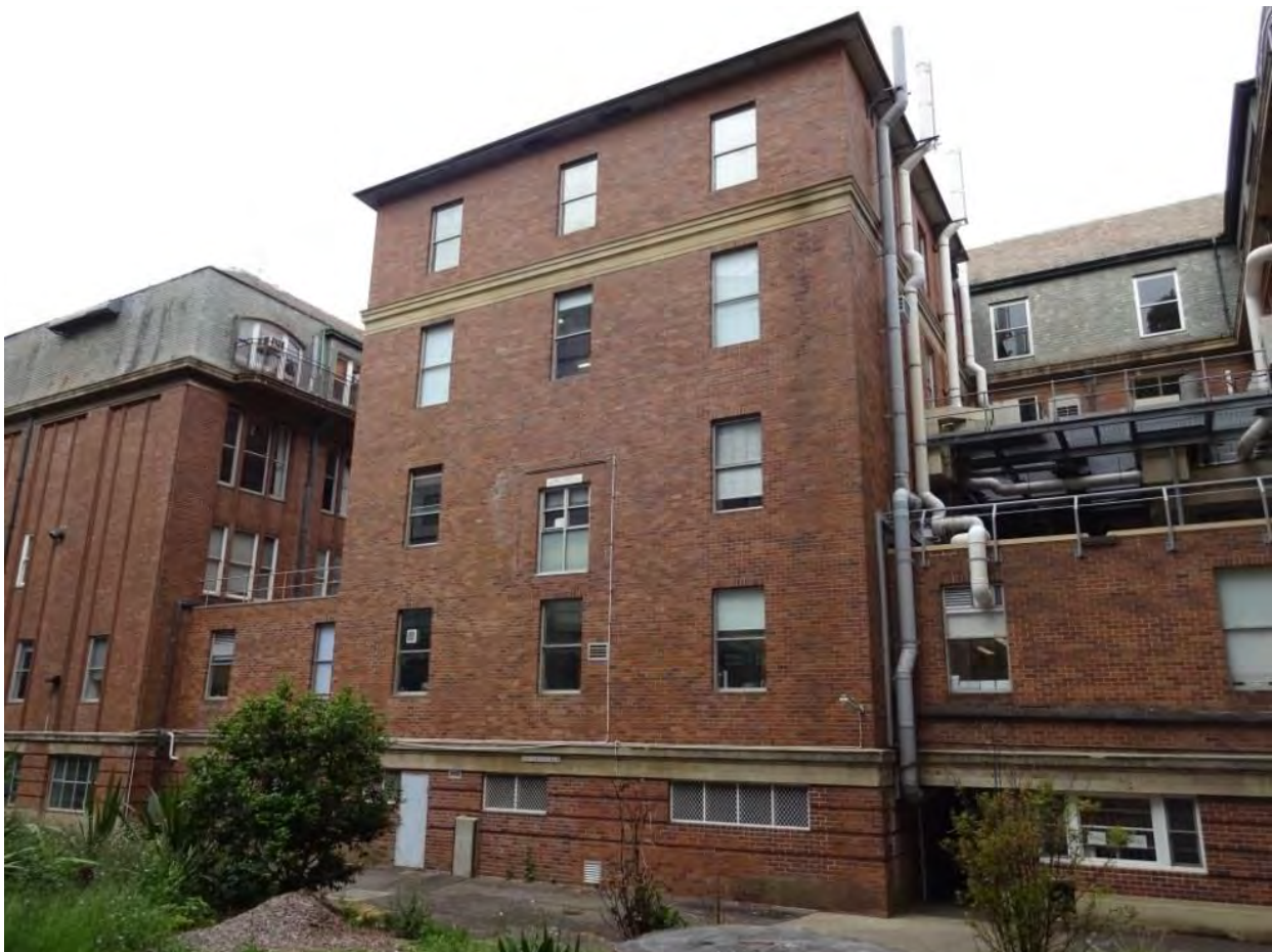
Figure 5 – View of the rear (western) façade of the building
