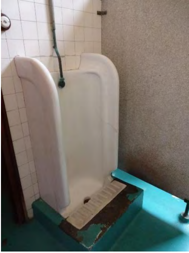
Picture 15 – Art Deco urinal – level 4 men’s WC (434)
