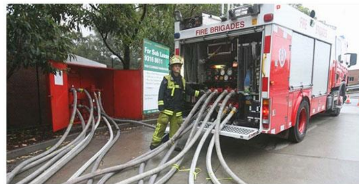
A fire engine connecting to the fire booster assembly in the event of a fire.
