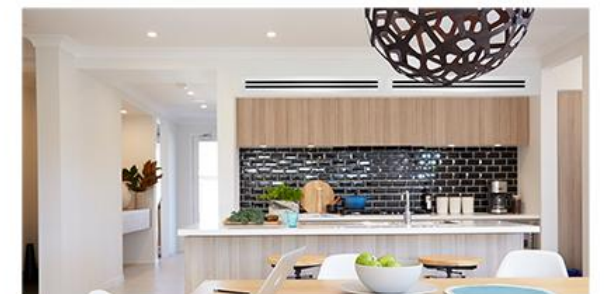
Supply grilles within the kitchen joinery
