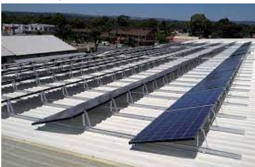
Tip: Angled at 30 degrees as shown and ideally north facing located in an area with no over shadowing from surrounding buildings/structures/planting
