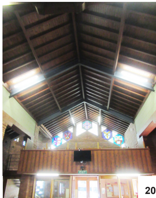
16 View of Church from south-east 18 Protruding key bricks, southern facade 20 View west in Church, showing gallery, steel rafters and green acoustic panels
