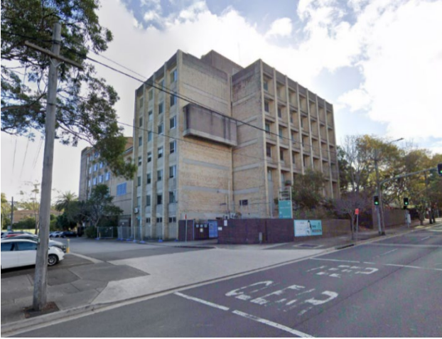
TAFE Bankstown, located further north of the site
