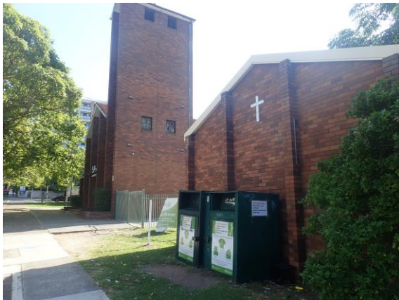
Figure 5.1 St Paul's Anglican Church, view to the north.
