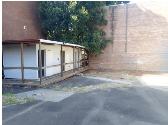
Figure 5.6 Area of hardstand with amenities block.
