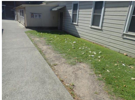
Figure 5.2 Area of ground surface exposure.
