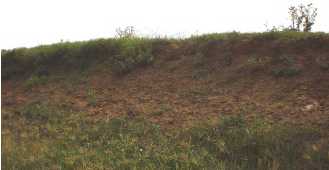
Photo 3 - Embankment located within Tranche 8
