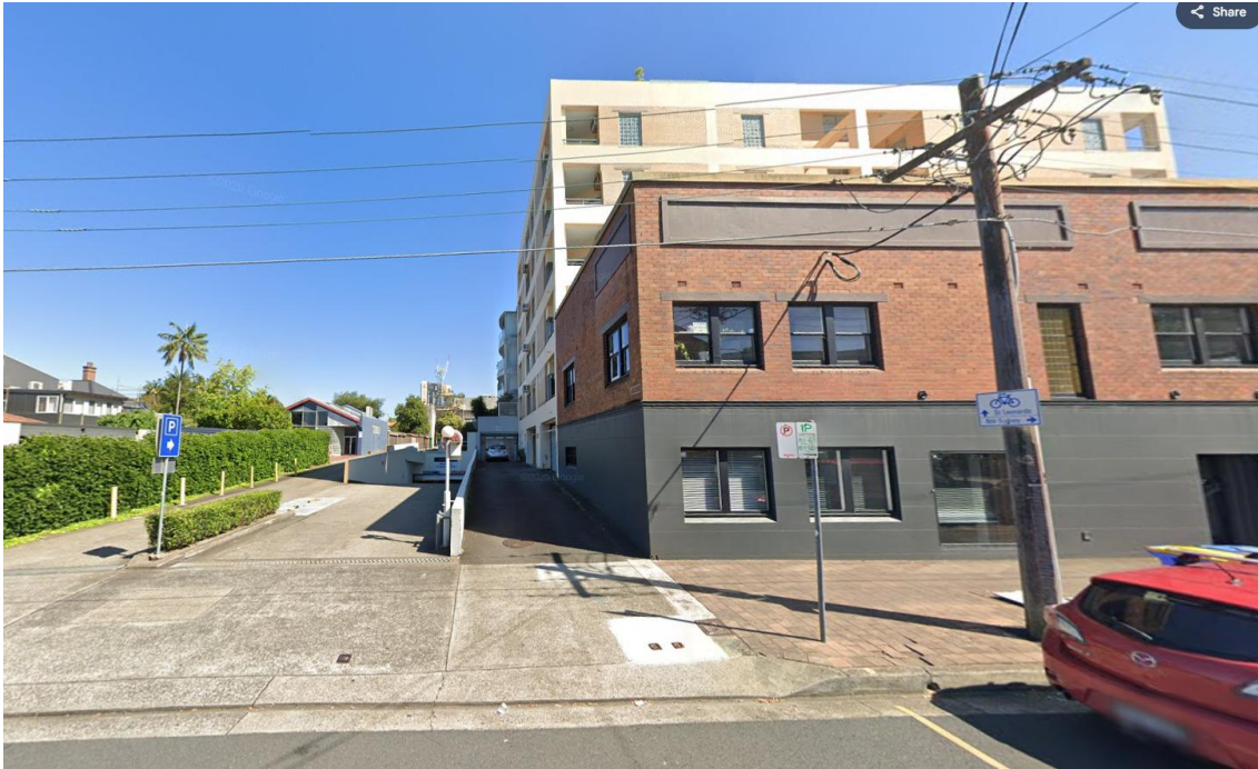
Figure 4: Existing development on the site viewed from Bruce Street (Source: Google Maps)
