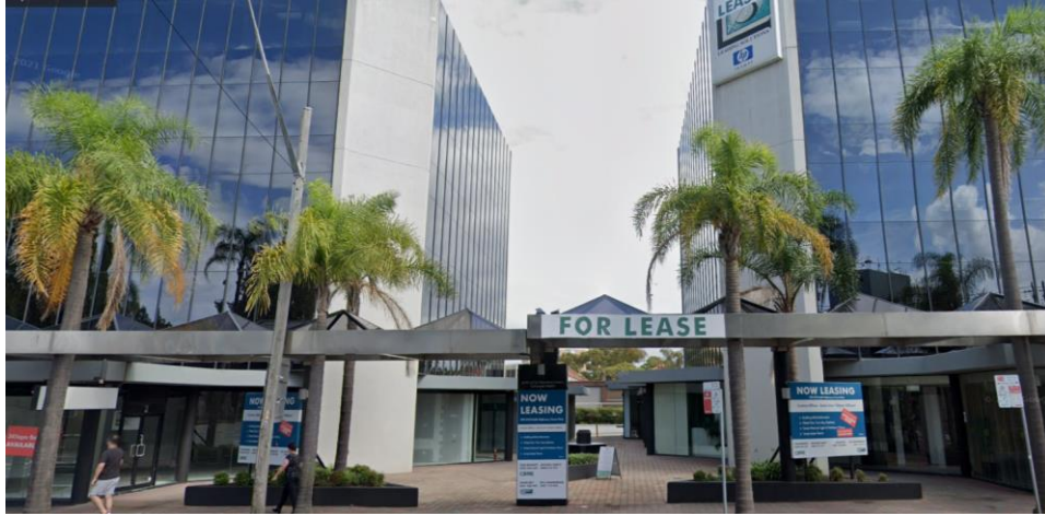
Photograph 1 – The site comprising two commercial buildings.
