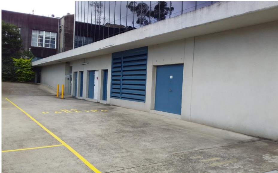
Photograph 2 – Storage rooms located at the rear of premises 272 Pacific Highway (on ground level).
