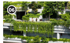
06 Podium Roof Planter
