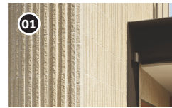
01 Ground Floor Facade Grc Cladding With Fluted Grooves In Soft Sandstone Finish
