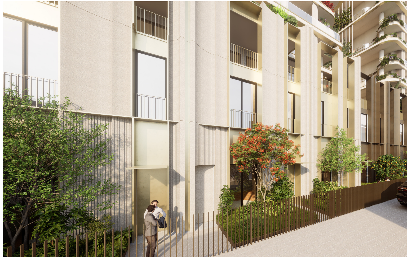
03 Podium Facade Reveal Aluminium Facade Cladding And Steel Awning In Light Bronze Finish
