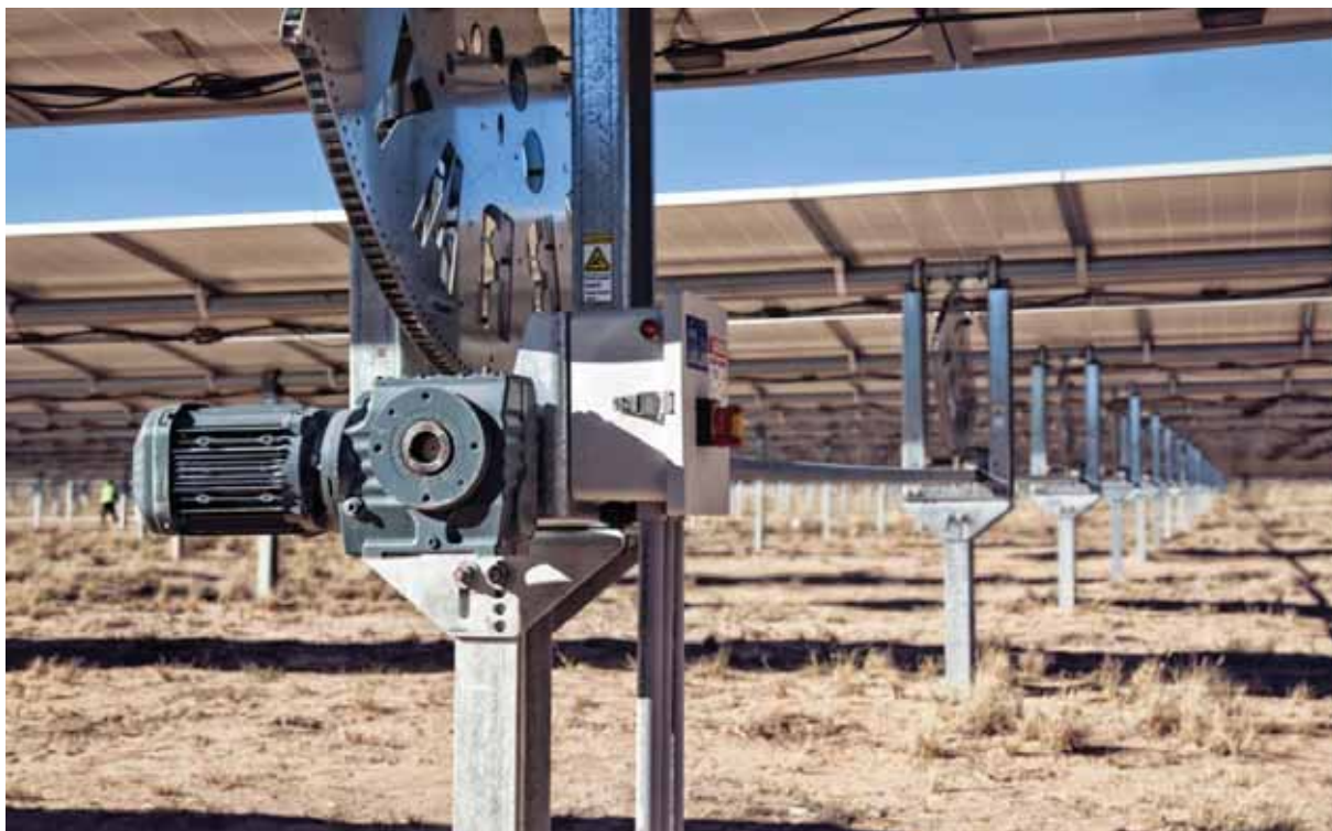
Photograph 3.2 Example of the steel frame structures used to support PV solar panels
