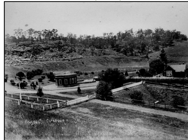
Figure 9: Prospect Reservoir showing lower valve house c.1888 23
