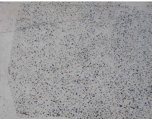
PV01: INSITU CONCRETE PAVING, EXPOSED AGGREGATE
