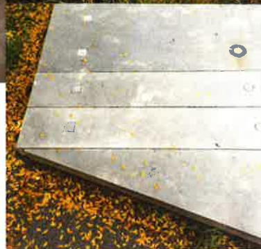
PRECAST CONCRETE (LAGOON PERIMETER)
