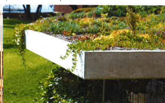
SUSPENDED SLAB GREEN ROOF (CURVED AWNINGS)
