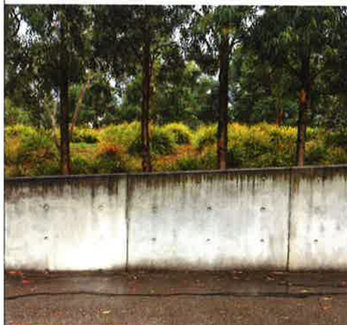
INSITU CONCRETE (RETAINING)
