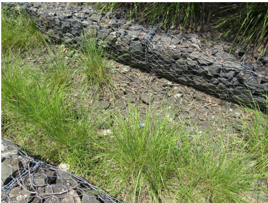
Figure 30 PHOTO POINT 3 – PARTIALLY VEGETATED GABION SWALE
