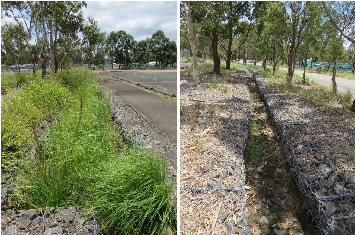
Figure 29 (LEFT) PHOTO POINT 1 - VEGETATED GABION SWALE, (RIGHT) PHOTO POINT 2 - UNVEGETATED GABION SWALE
