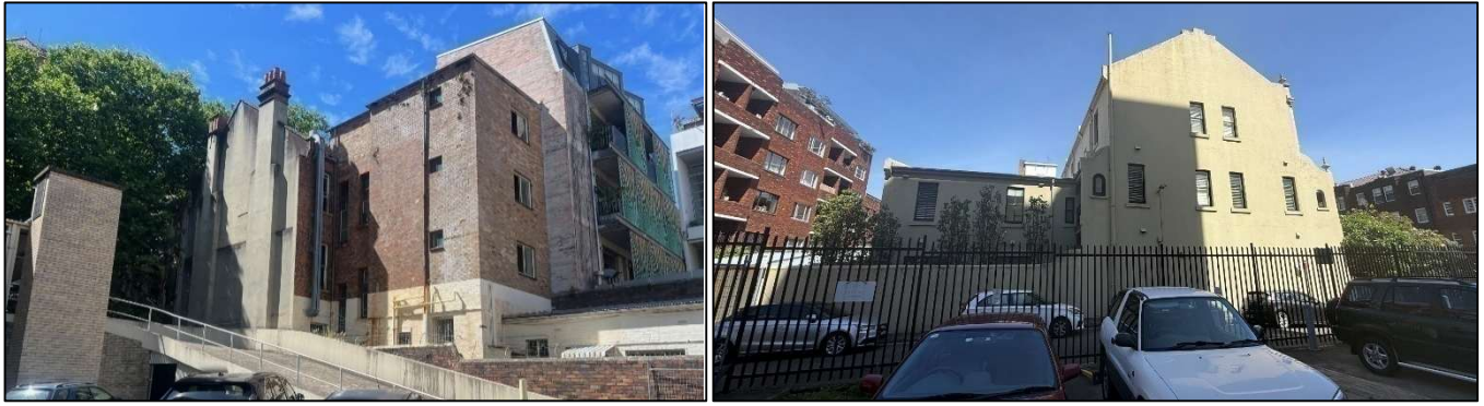
Figure 11 | Northern elevation of 55 Macleay Street (left) and western elevation of 9 McDonald Street (Source: DPHI)
