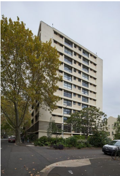
Picture 1 View from North (Macleay Street)
