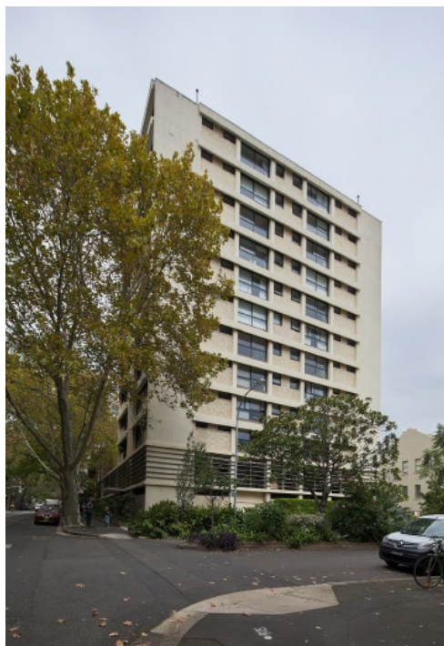
Picture 1 View from North (Macleay Street)
