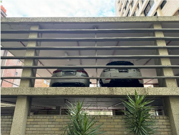
Picture 1 Existing carpark
