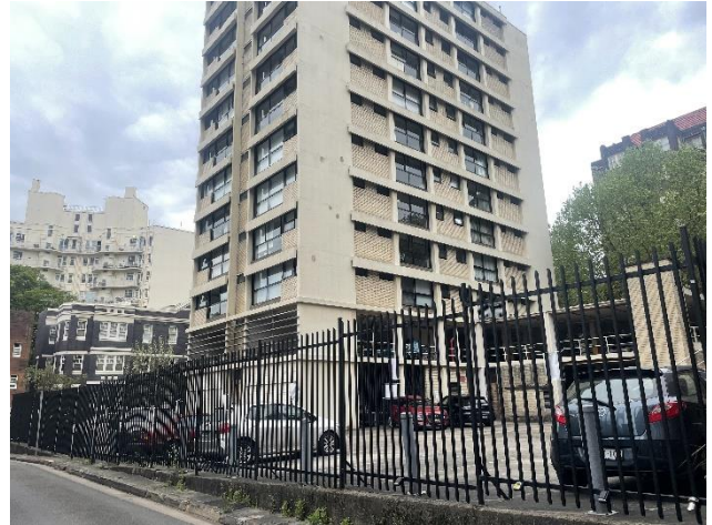
Picture 2 View of site from Mc Donald Street, facing south east
