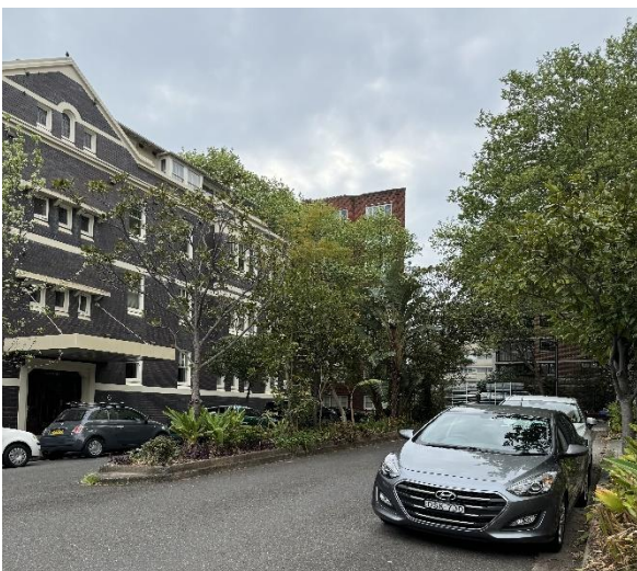
Picture 5 Dead end on McDonald Street, facing north
