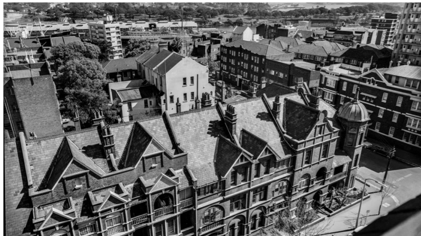
2. 45-53 Macleay Street site August 1962 (Source: City of Sydney Archives)
