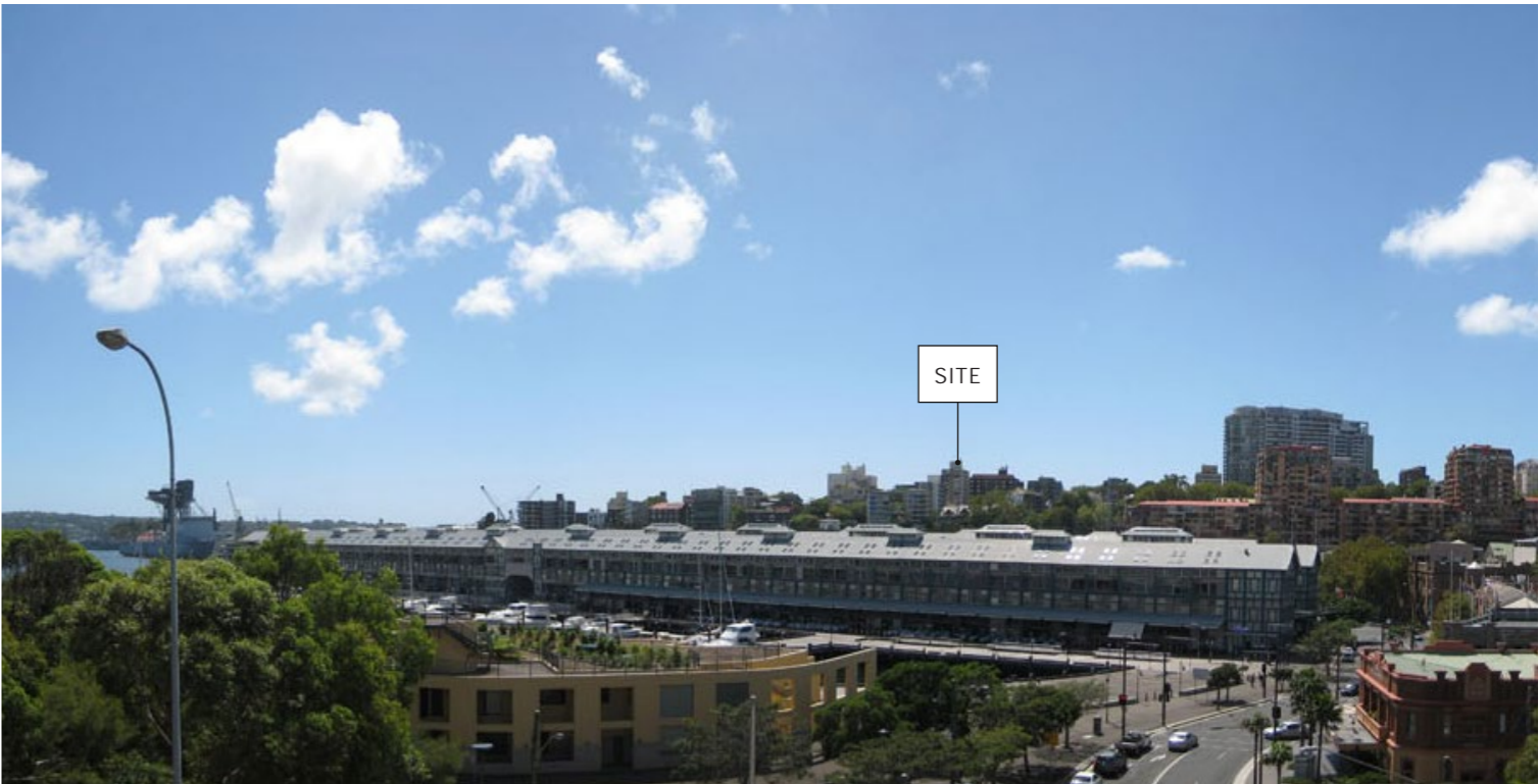
Contribution of existing building to Potts Point ridgeline
