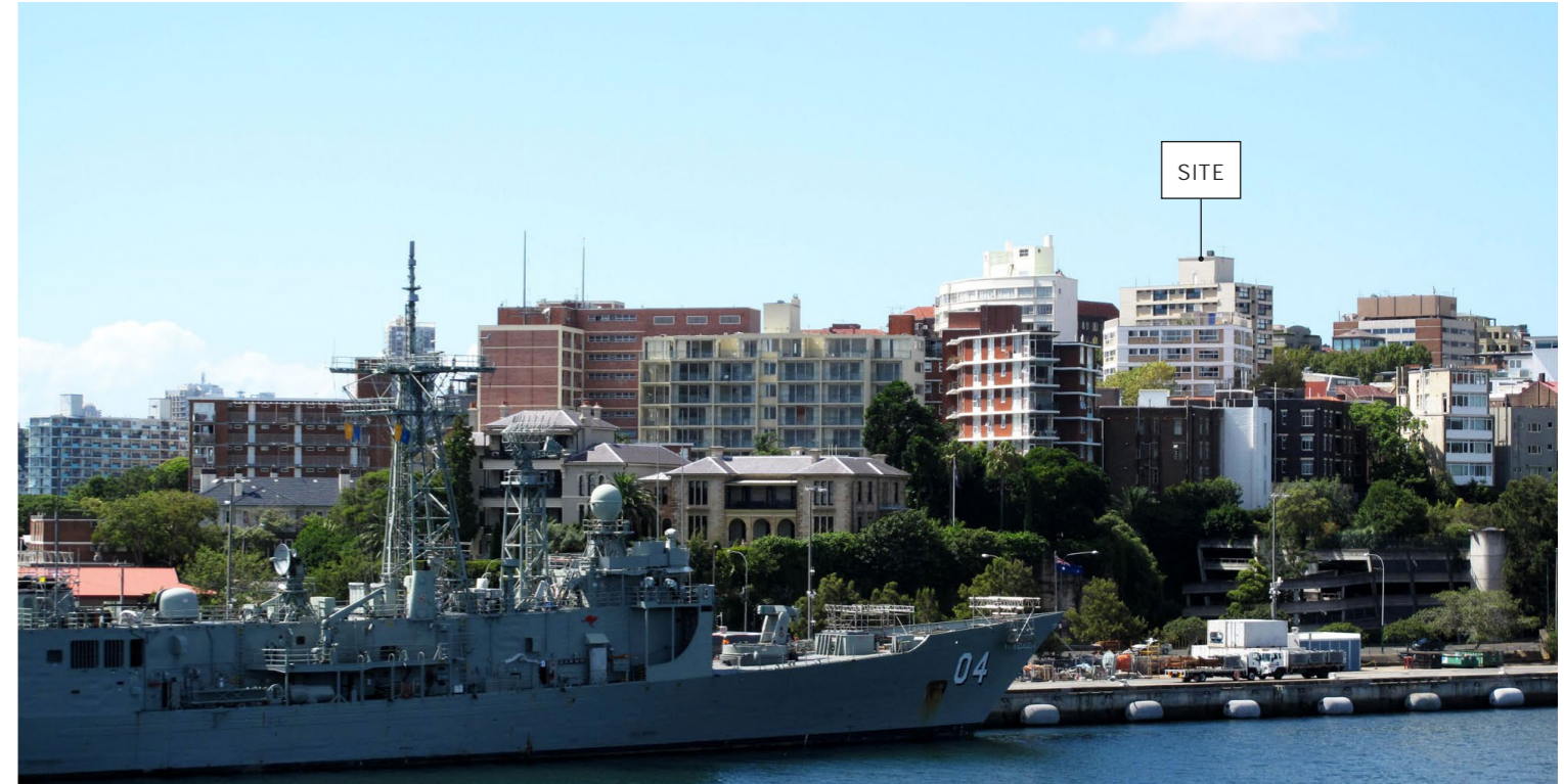
Contribution of existing building to Potts Point ridgeline
