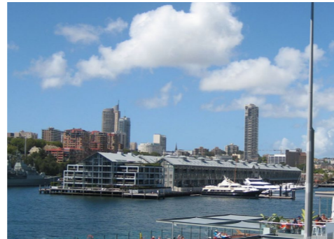
2. Woolloomooloo Finger Wharf (I1)
