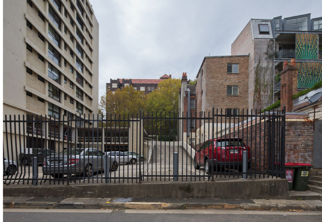
View to rear of site from McDonald Lane
