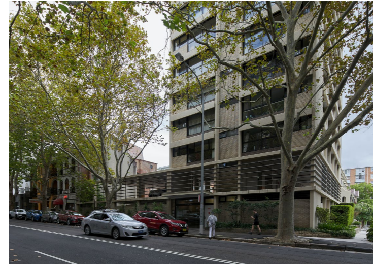
Existing site condition with car parking to Ground and Level 1
