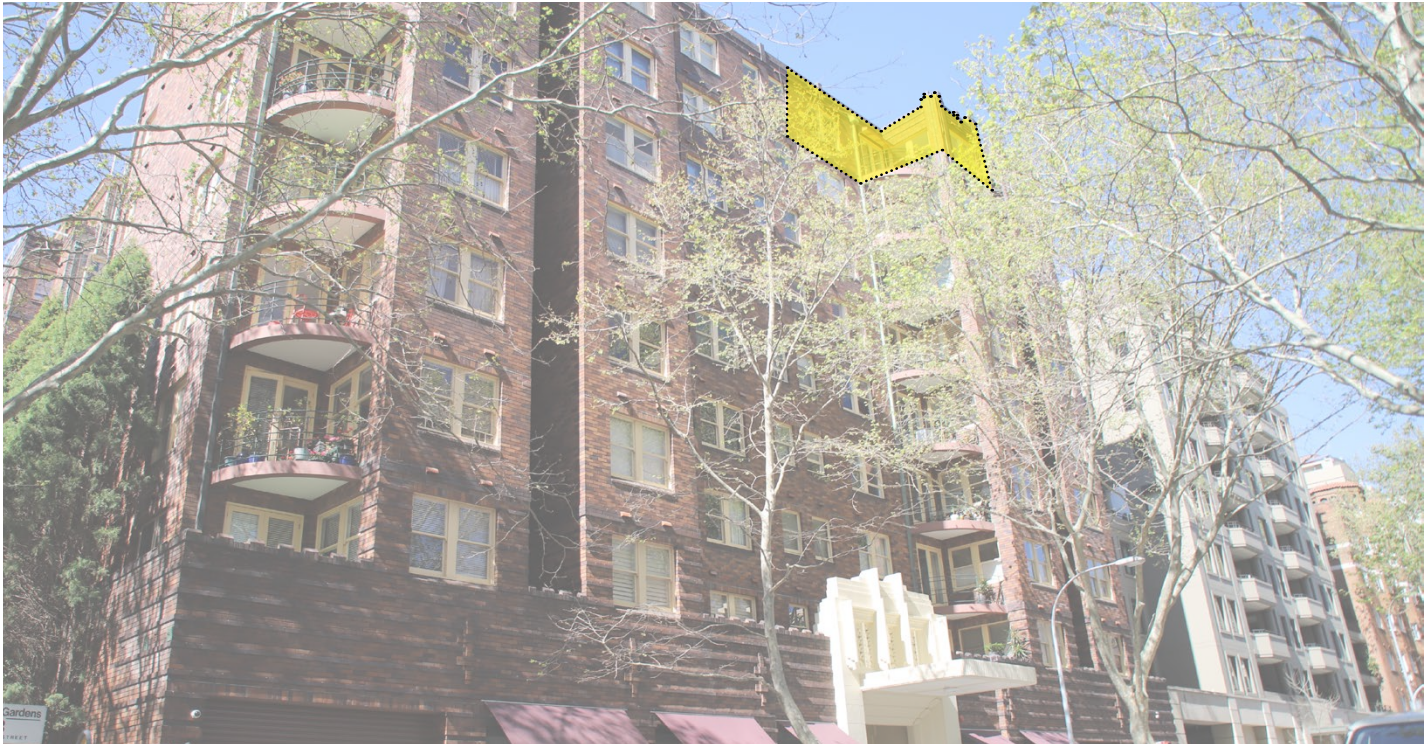
Figure 23 Macleay Regis eastern elevation, location of Unit 203 indicated in yellow.
