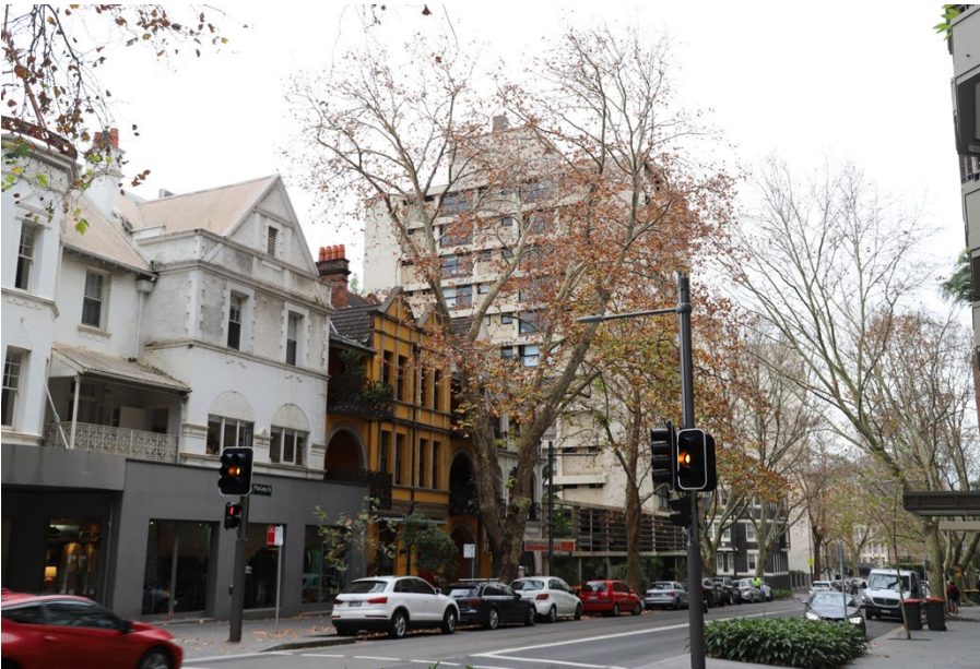
Figure 20 Streetscape detail of 55 (adjacent to site) and 57-59 Macleay Street (Yellow House).
