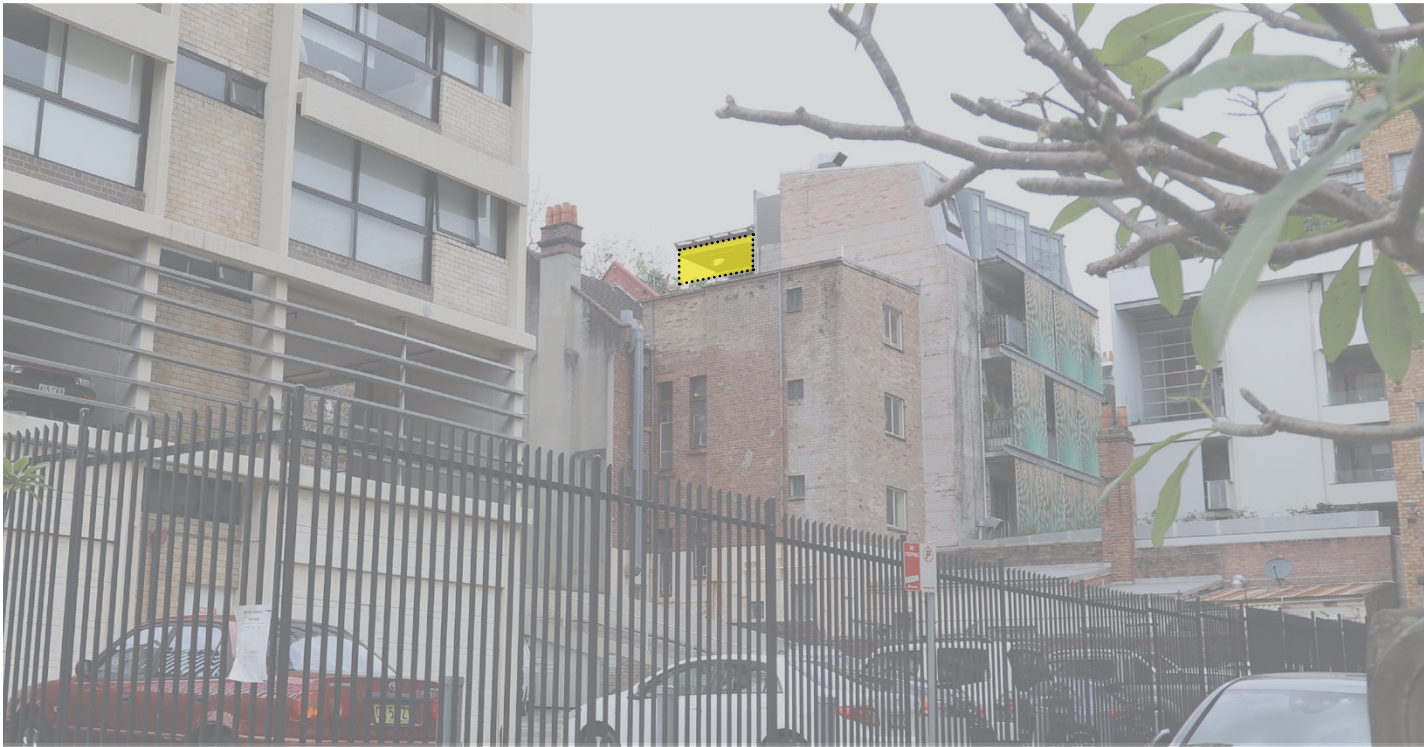
Figure 28 Rear view of Yellow House from McDonald Street towards northern elevation of building, location of Unit 7 balcony indicated in yellow.
