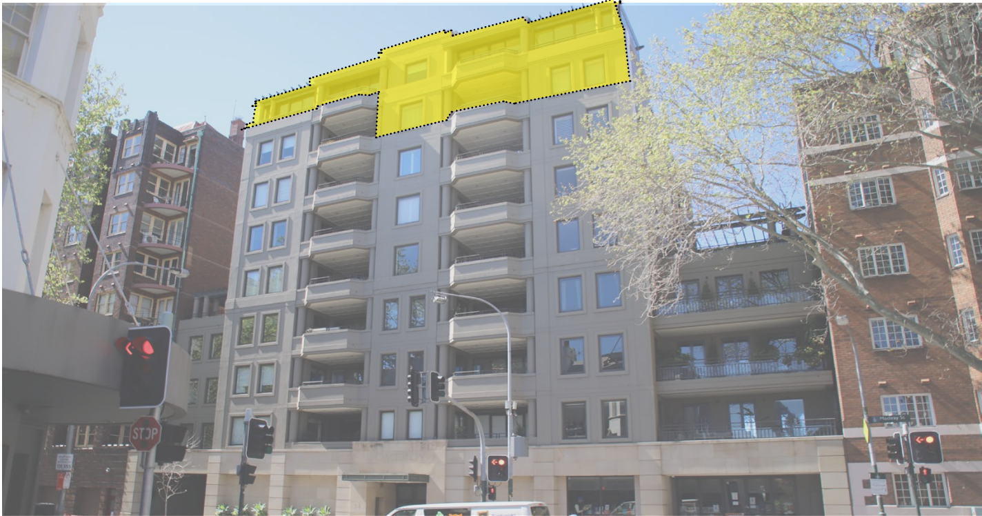
Figure 28 Macleay Regis eastern elevation, location of Unit 801 indicated in yellow.
