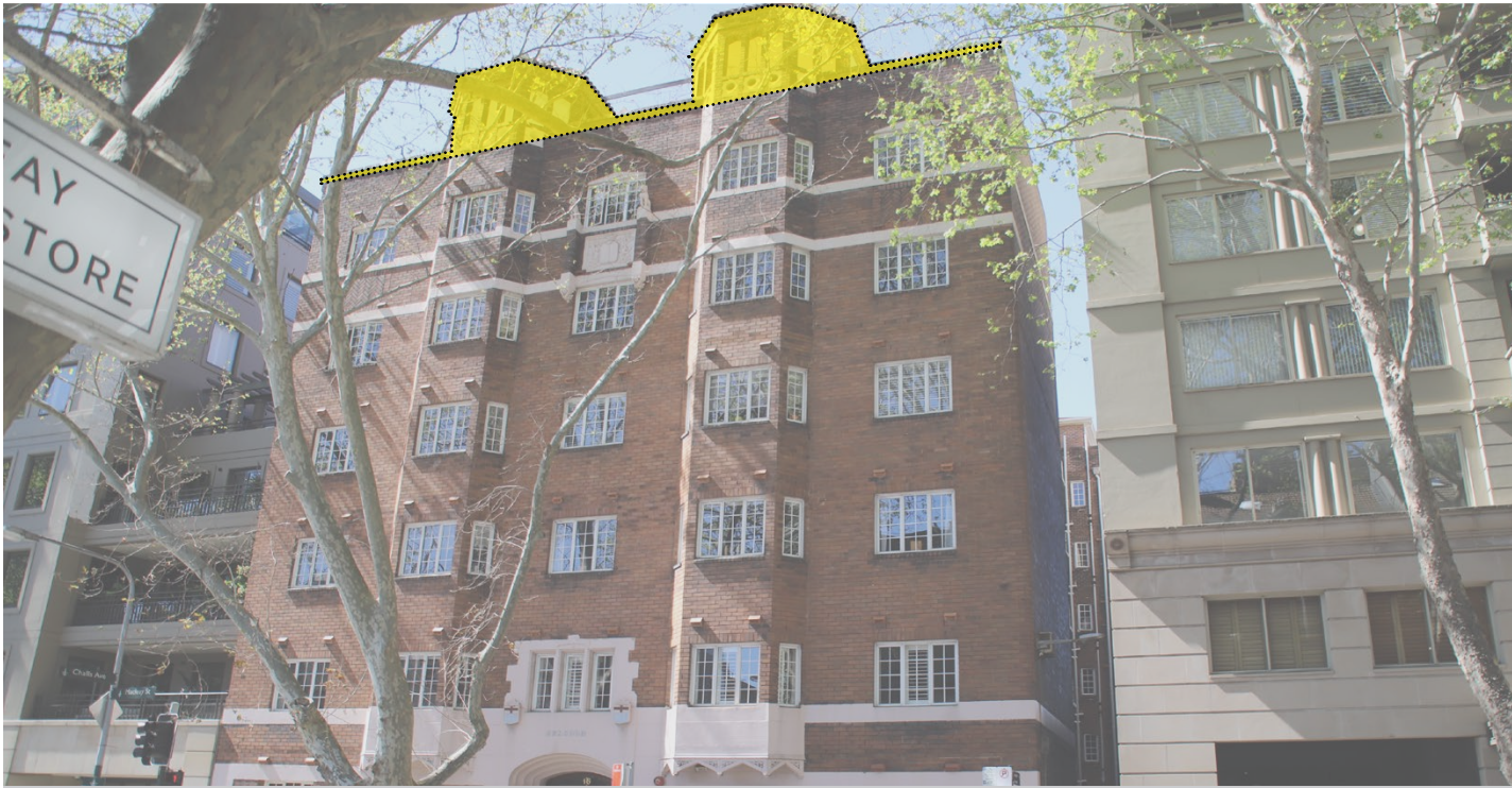
Figure 28 Eastern elevation of Selsdon location of Unit 60 roof terrace indicated in yellow.
